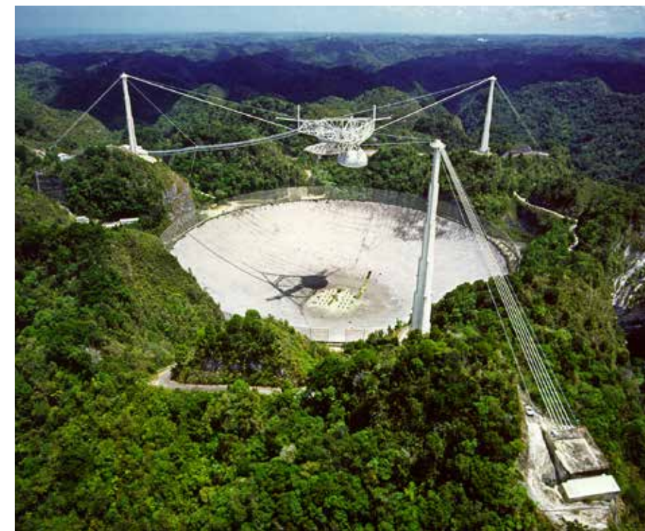
The Arecibo Observatory in Puerto Rico is an important tool for finding pulsars. Astronomers use this 1,000-foot-wide (305 meters) radio telescope to scan the skies to locate more of these compact objects. Photo courtesy of the NAIC - Arecibo Observatory, a facility of the NSF
